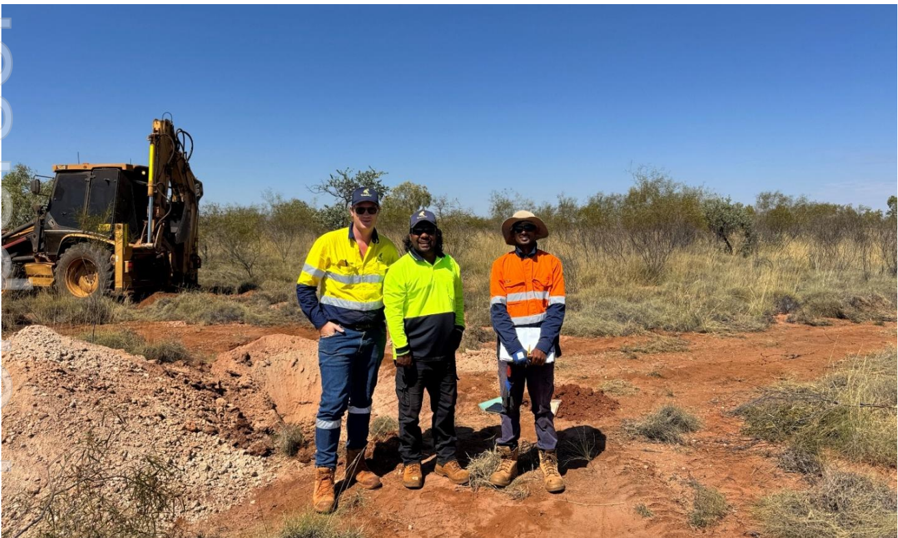
Plate 1 – Mike Dwyer (Wildcat Principal – Project Manager), Troy Eaton Jr (Nyamal Traditional Owner) and Alex Mathew (GALT Geotechnical Engineer) at a geotechnical test pit site within the NPI Area
