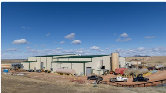
Central Processing Plant (Phase I & II)
