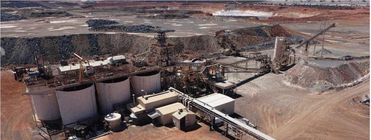
Figure 6. Kirkalocka Plant and ROM Pad with Kirkalocka open pit in the background (operated by Gylden Resources Pty Ltd)
