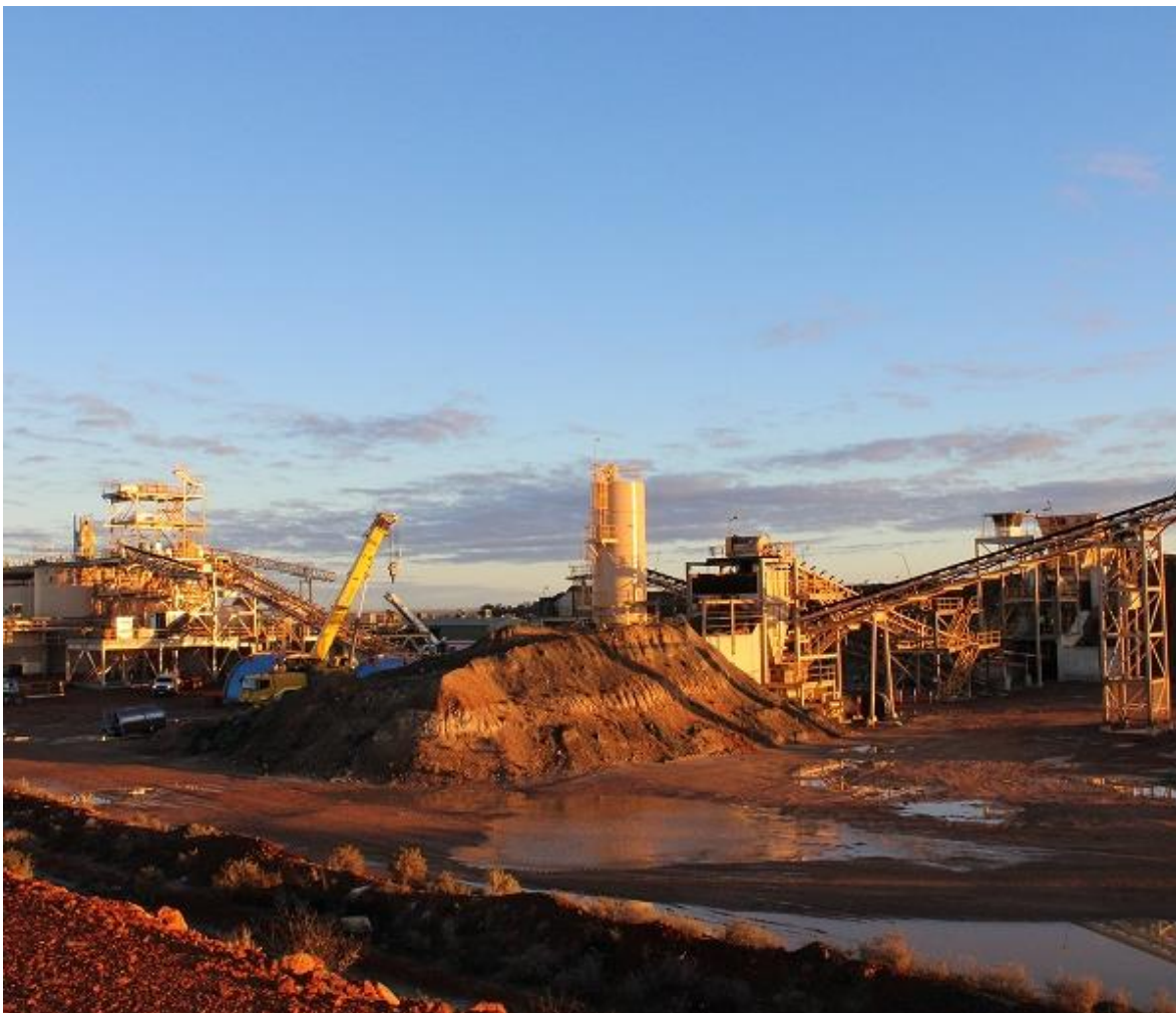
Figure 1. Kirkalocka Gold Processing Plant (operated by Gylden Resources Pty Ltd)
