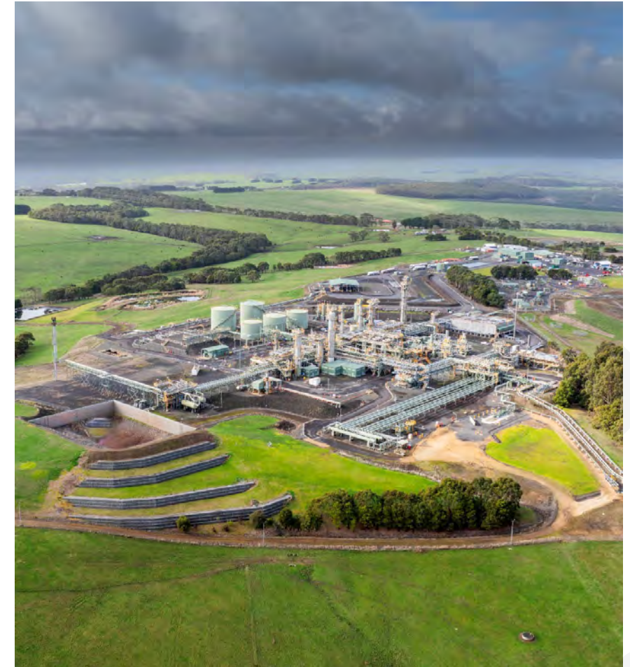
Otway Gas Plant
