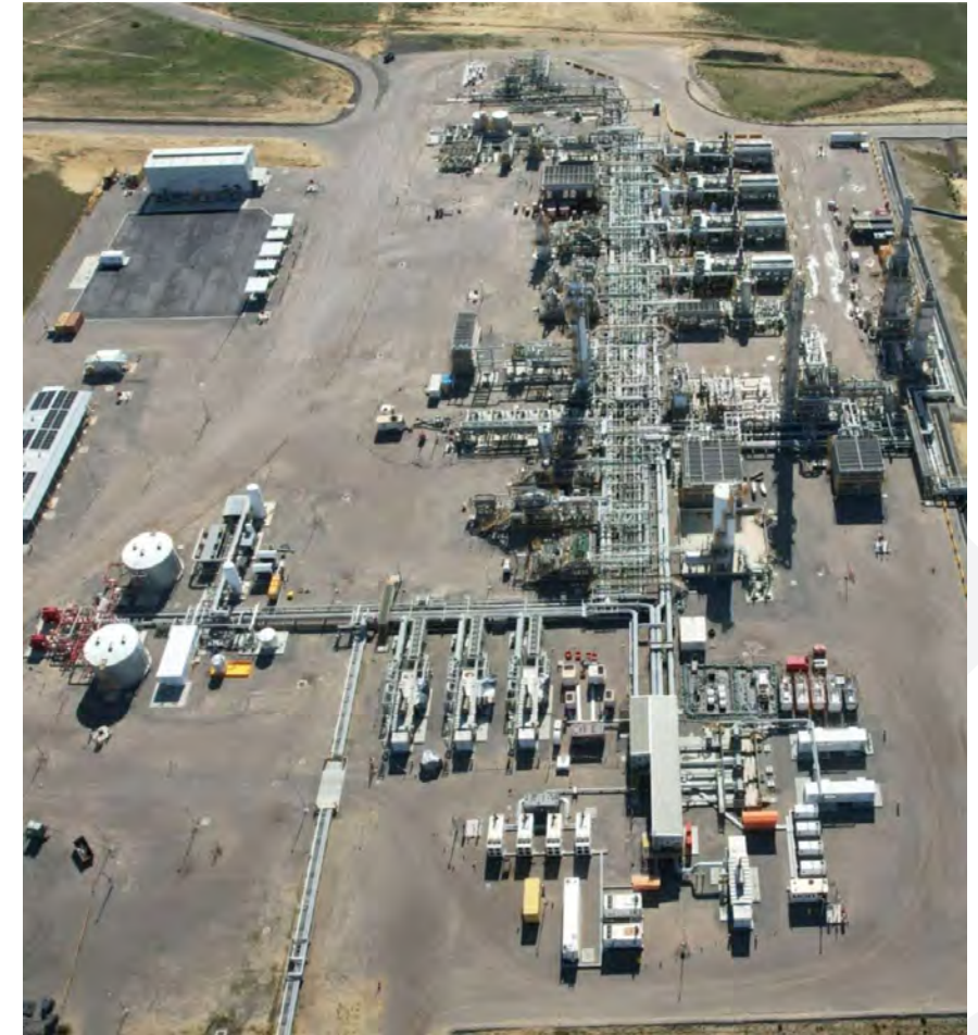
Waitsia Gas Plant
