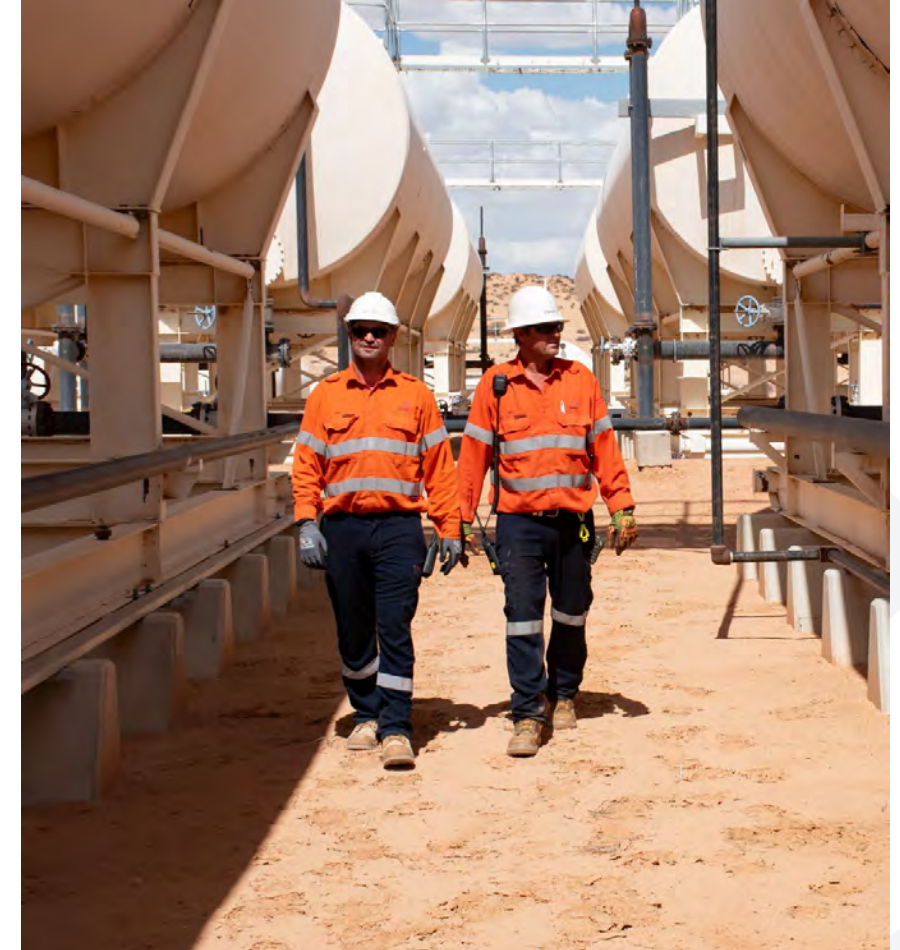
Western Flank, Bauer North Tank Farm
