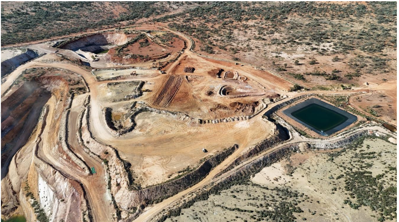
Figure 2 - Site remediation works underway in preparation for construction to commence
