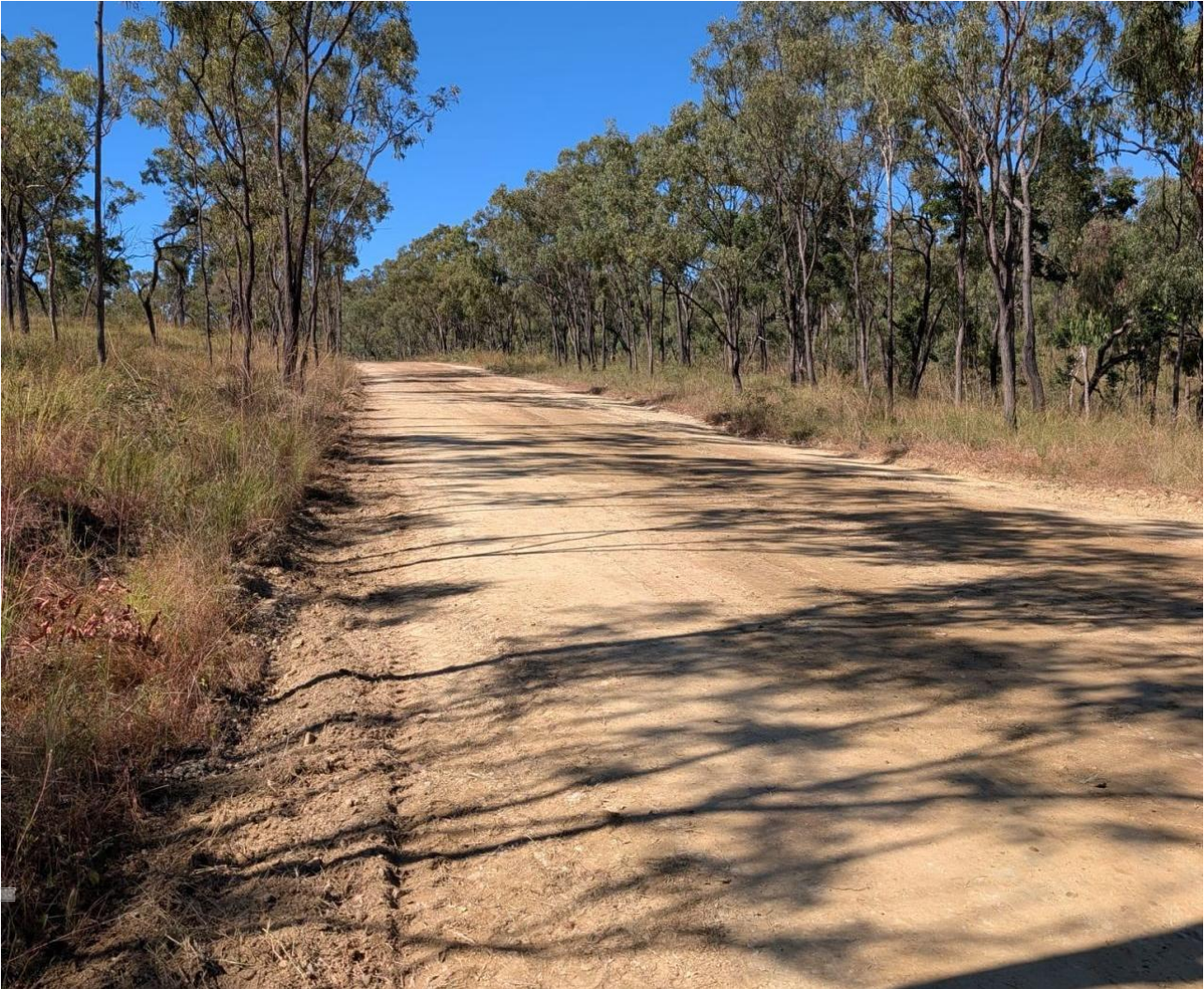
Figure 1: Dianne Copper Mine Project site access road
