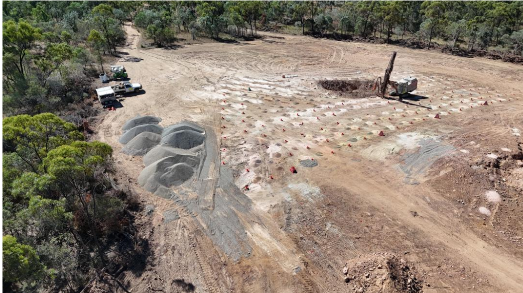
Figure 8: 277.5-004 Drill & Blast activities ongoing as part of second blast scheduled later in the month.
