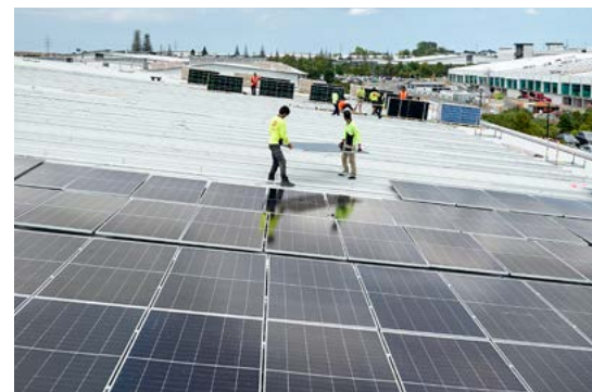
ROOFTOP SOLAR PANELS BEING INSTALLED AT OUR EAST TĀMAKI, NEW ZEALAND CAMPUS IN THE 2026 FINANCIAL YEAR.
