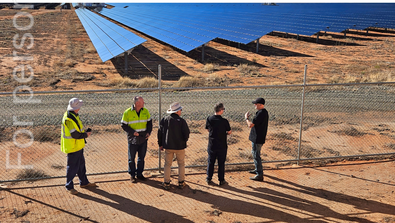
Image 6 Broken Hill 53MW Solar Farm
