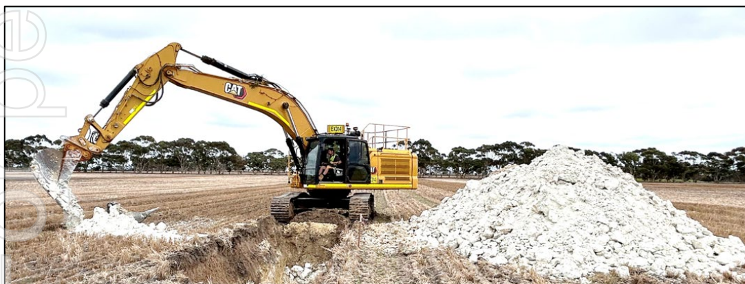
Test Pit GKTP007 Excavation – White Swan Kaolin Project, May 2026
