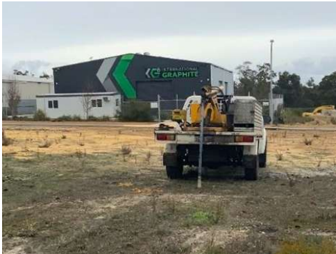
Left: Geotechnical drilling on site.
