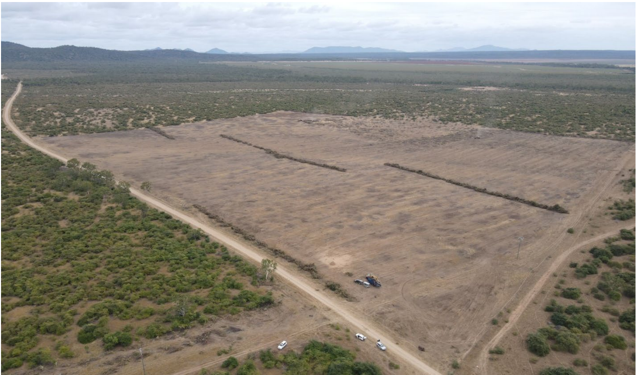
Aerial shot of project site post clearing and preparation of feedstock into windrows
