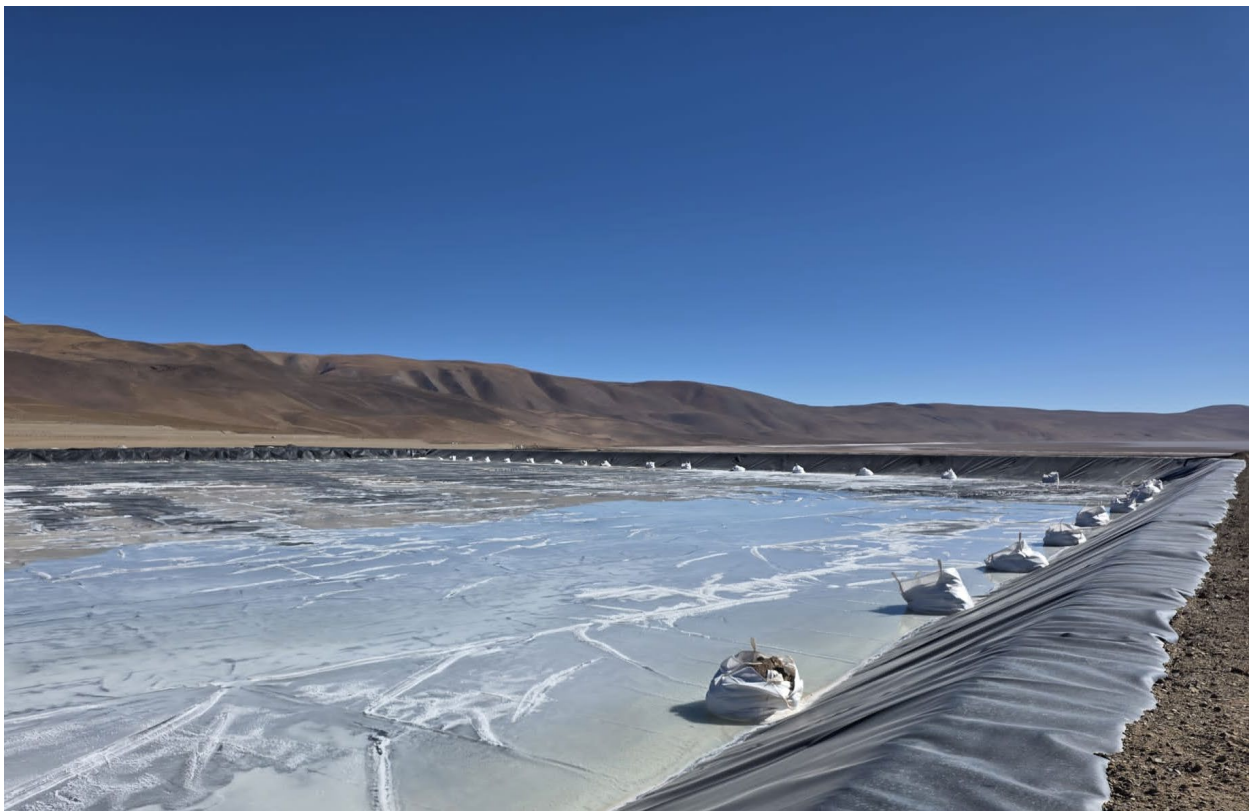
Figure 1. Processed brine discharged into final evaporation pond.
