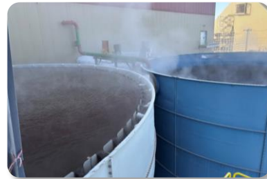
Thickener and process water tanks
