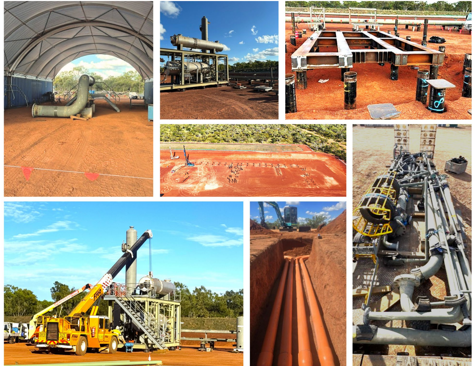
On-site installation of the Carpentaria Gas Plant is underway
