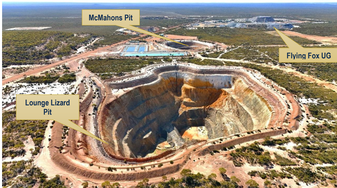
Figure 5: Aerial view of Lounge Lizard pit and McMahon's pit
