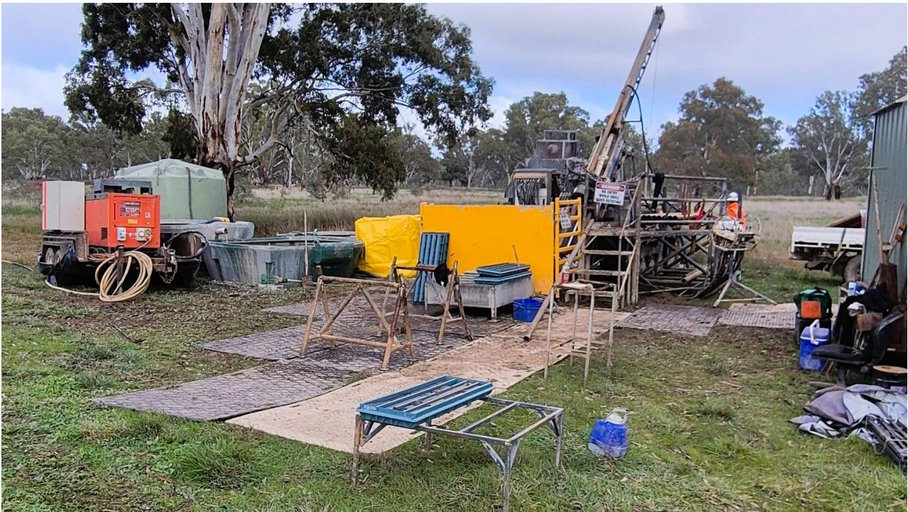
Drill rig drilling east from the west end of the West Pit (3 June 2026)
