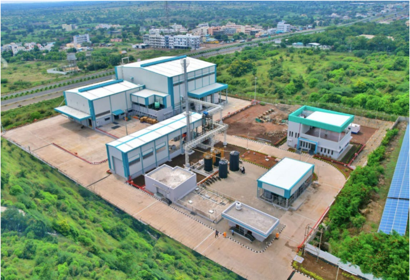
Expandable Graphite JV Facility near Pune, India
