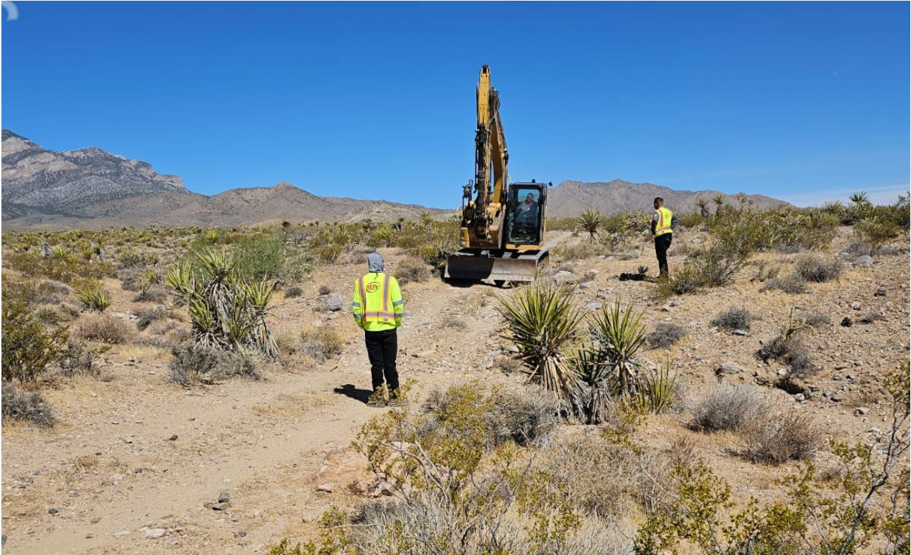
Figure 5: Access track upgrade works at Desert Star
