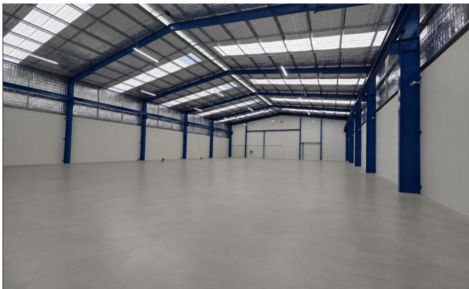
Completed Factory Extension
