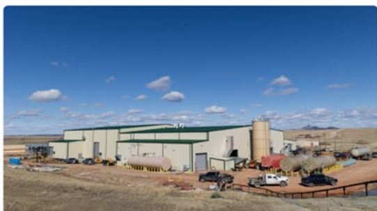
Central Processing Plant (Phase I & II)
