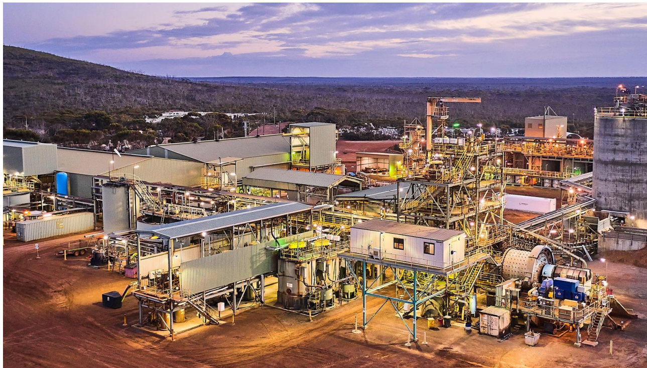
Figure 1: Existing CBC infrastructure with MREP plant and primary ball mill annotated
