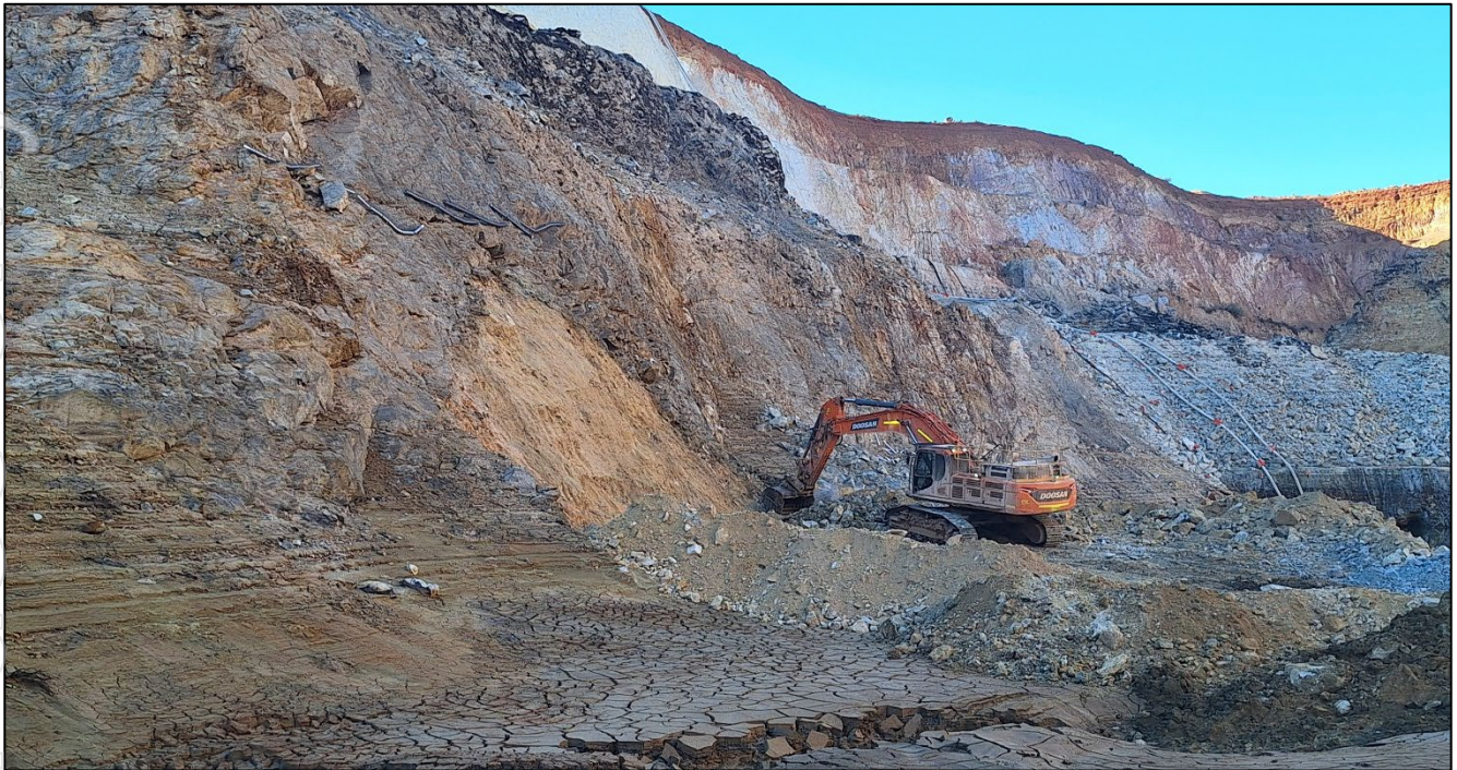
Figure 2 – Pollard Decline access preparation
