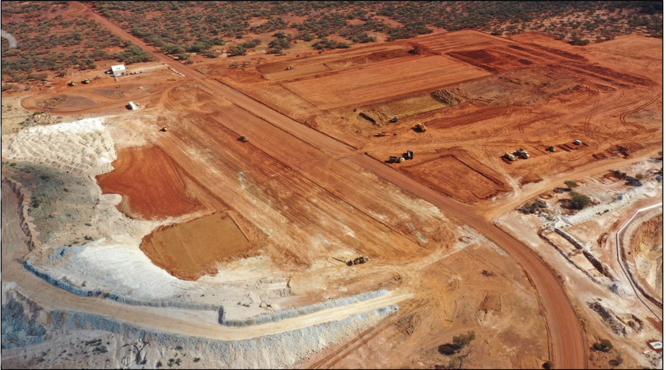
Figure 6 – Processing plant bulk earthworks nearing completion
