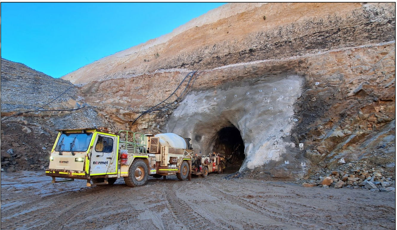
Figure 1 – Stripping at the Youanmi Decline
