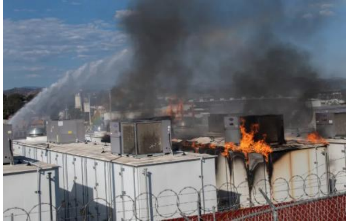
Escondido, California (September 2024): A BESS fire at a substation resulted in significant damage. The incident involved overheating of battery cells. Source: https://eticaag.com/thermal-runaway-in-battery-energy-storage-systems-bess/
