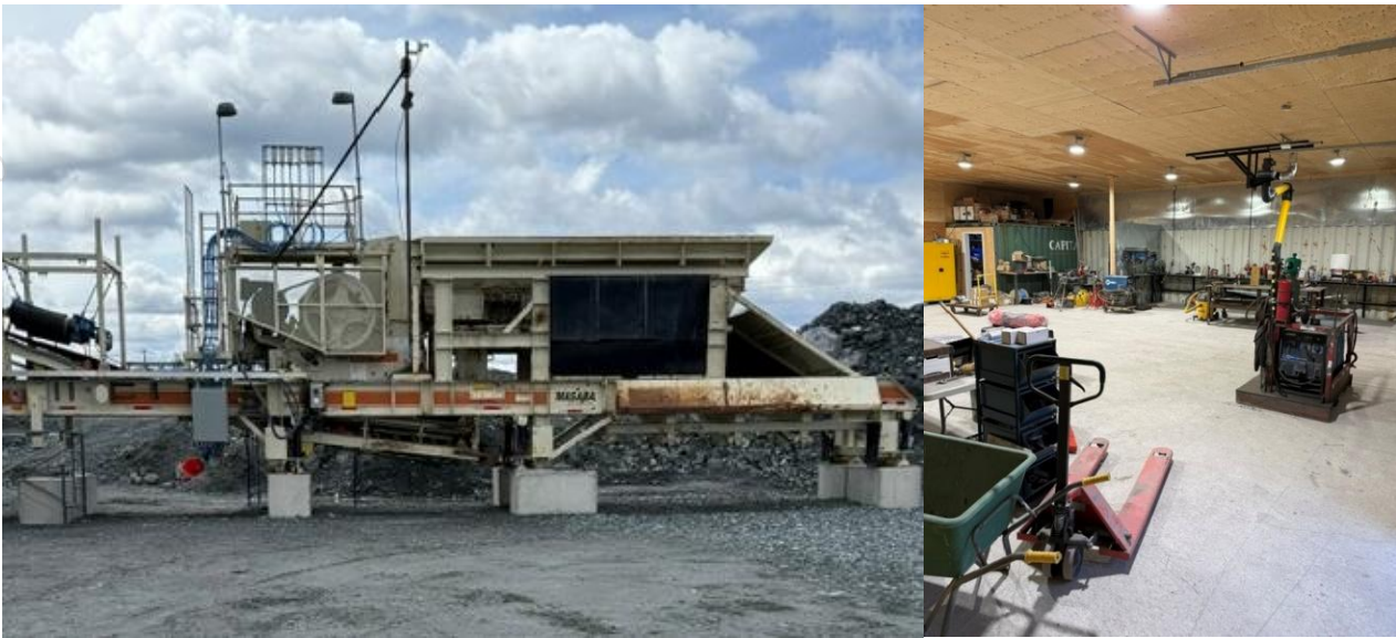
Figure 5: New crusher footings in place and inside of new mill maintenance workshop
