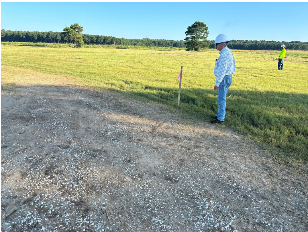
Figure 1: Site preparation activities at Zydeco-1
