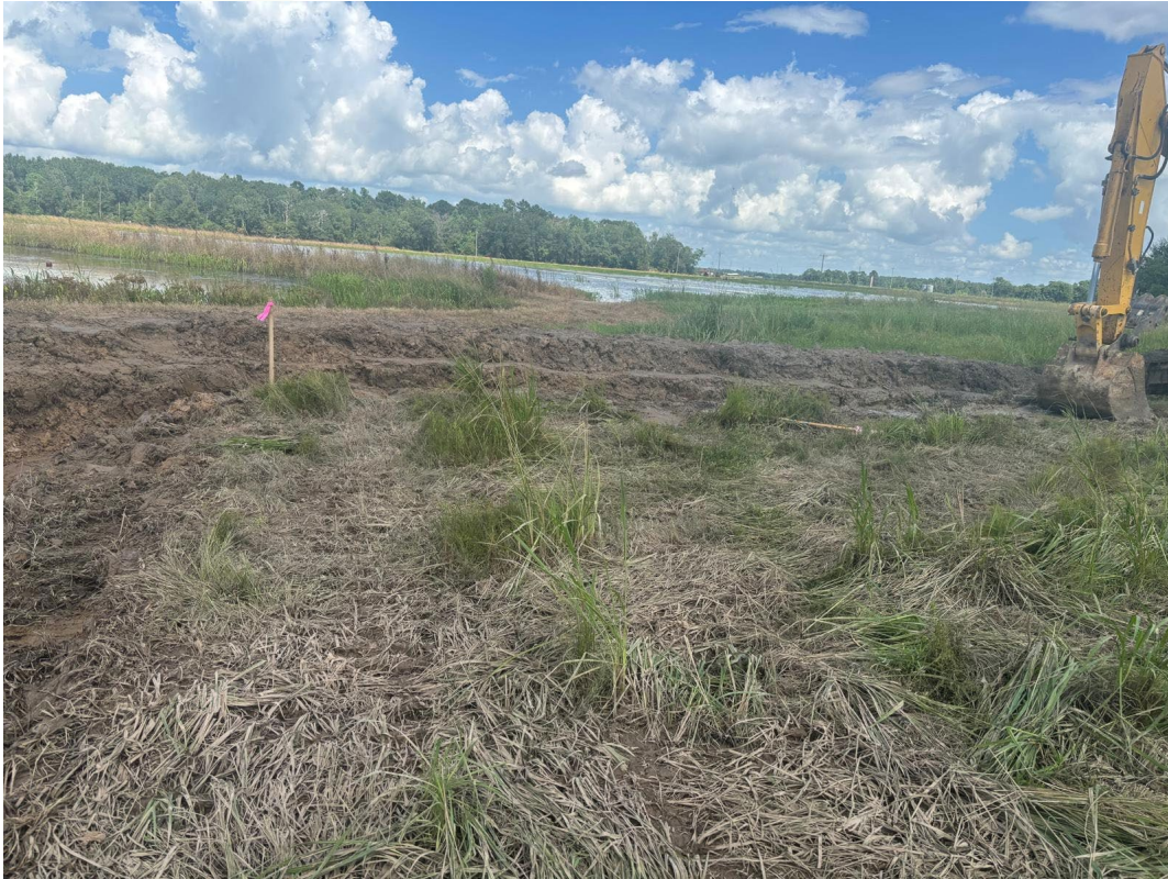
Figure 2: Drilling pad construction
