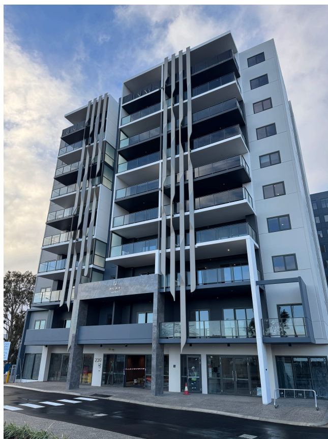
Figure 1. Bel-Air Apartments site photo, Belmont
