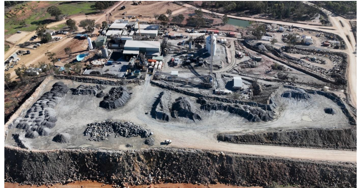
Figure: Mineral Hill ROM pad stockpile and processing plant (June 2026)
