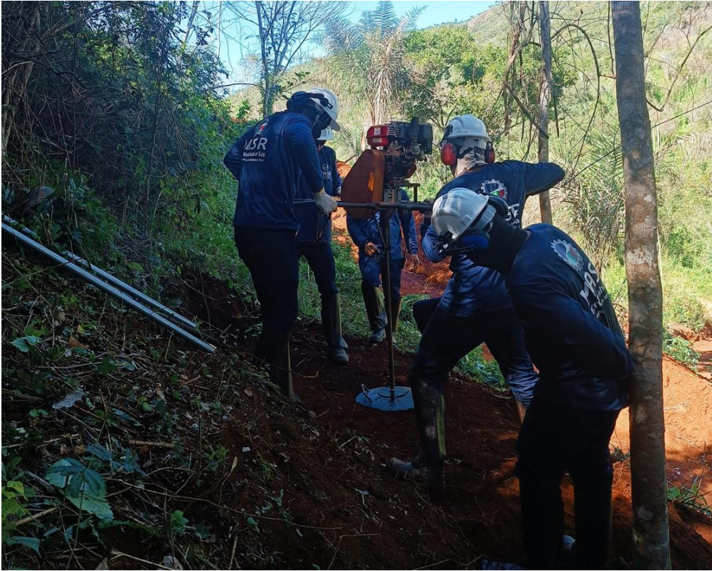
Figure 2: Drilling one of the first holes with the auger drill at one of the priority locations for the Campo Grande Project.
