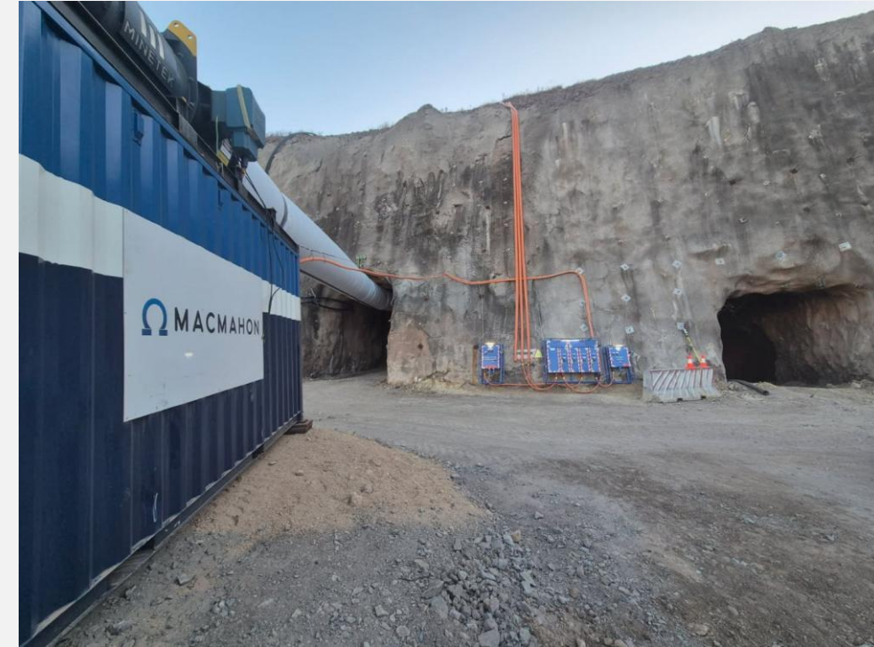
Underground operations at Mt Carlton
