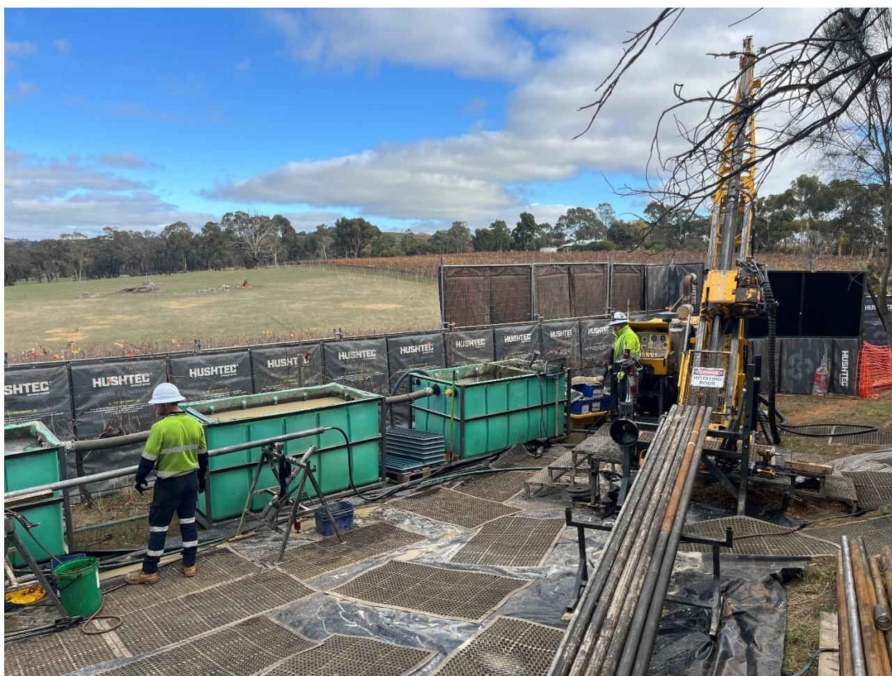
Figure 6 – Diamond drilling underway at the Irvine Gold Project north of the Resolution Lode. The rig is targeting one of the Exploration Target areas identified in the updated JORC Resource and Exploration Target Statement. Picture taken 9-June-2026.
