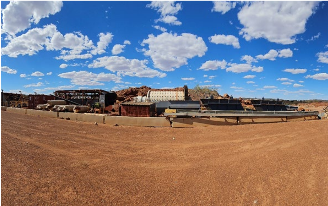
Figure 1: Ball Mill and associated plant
