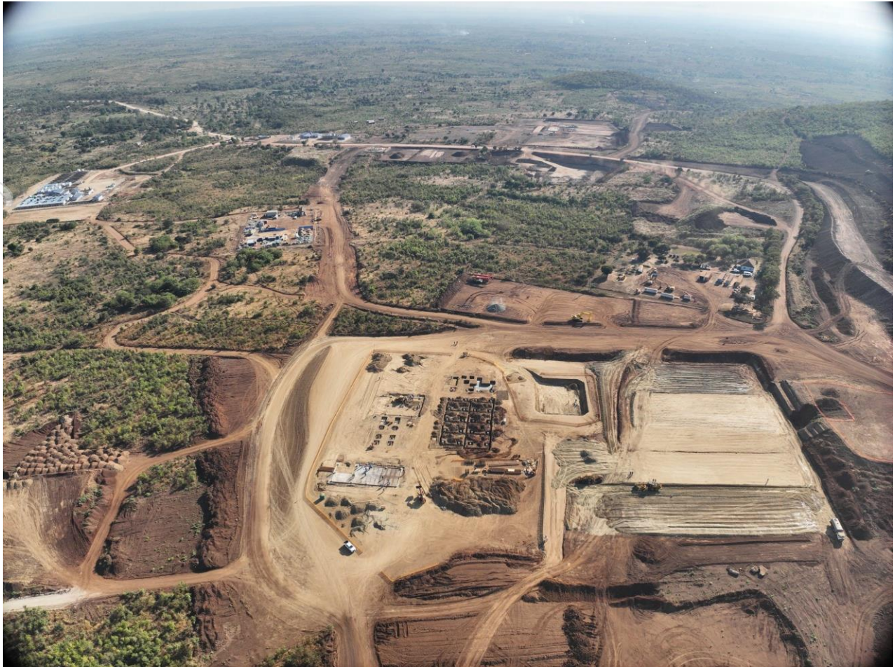
Picture 2. Overview of the Kangankunde process plant area, highlighting continued progress across civil works, earthworks and supporting infrastructure
