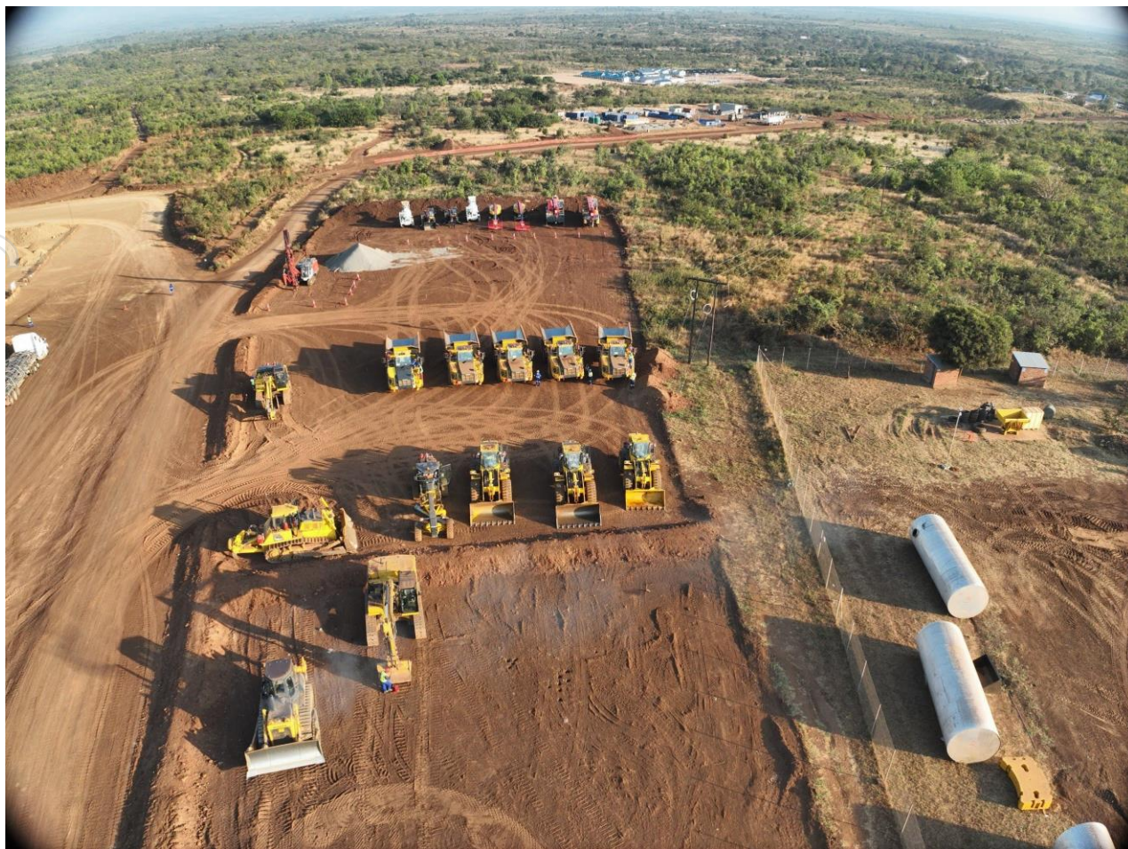
Picture 7. Kangankunde mining and infrastructure fleet
