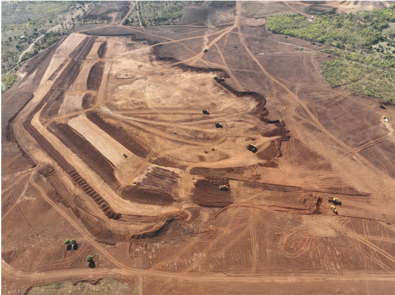
Picture 8. Kangankunde Tailings Storage Facility Progress
