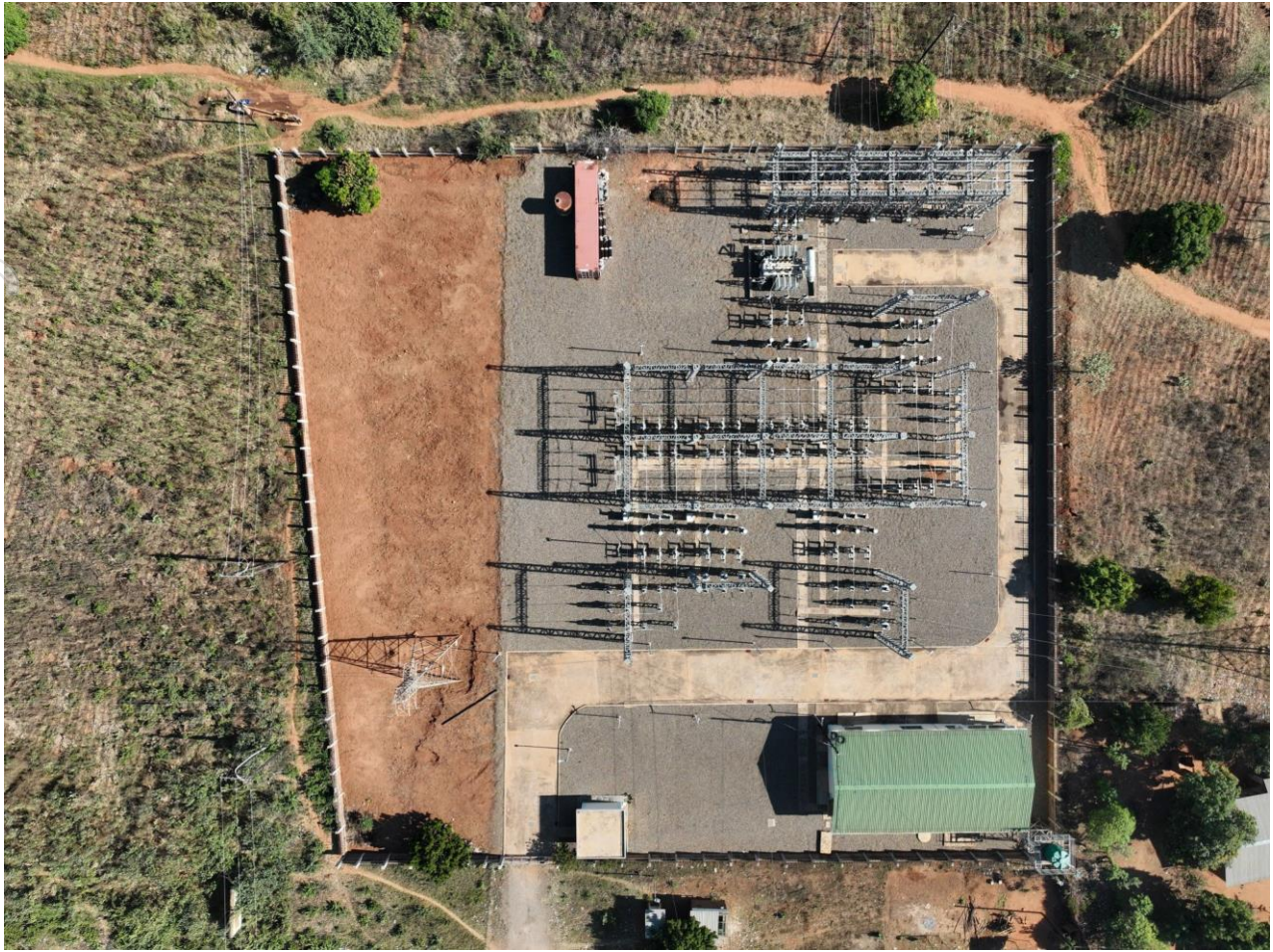
Picture 10. Balaka ESCOM substation tie-in point for the power corridor
