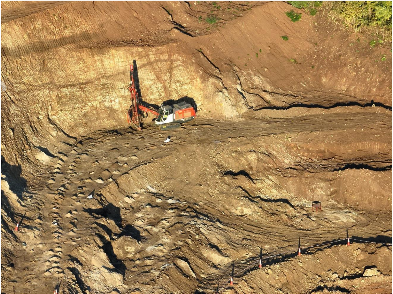
Picture 3. Production drill rig drilling the first blast pattern at the Stage 1 pit area, marking a key mining readiness milestone ahead of the planned first blast at Kangankunde
