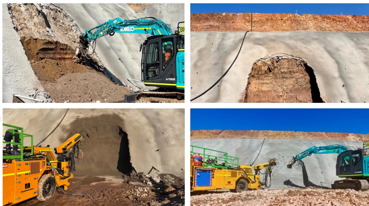
Figure 2: BP33 portal cut works (clockwise from top left): 1. Initial cut 2. Excavation of the portal completed 3. Fibrecrete applied to the face and brow 4. Fibrecreting of portal cut completed
