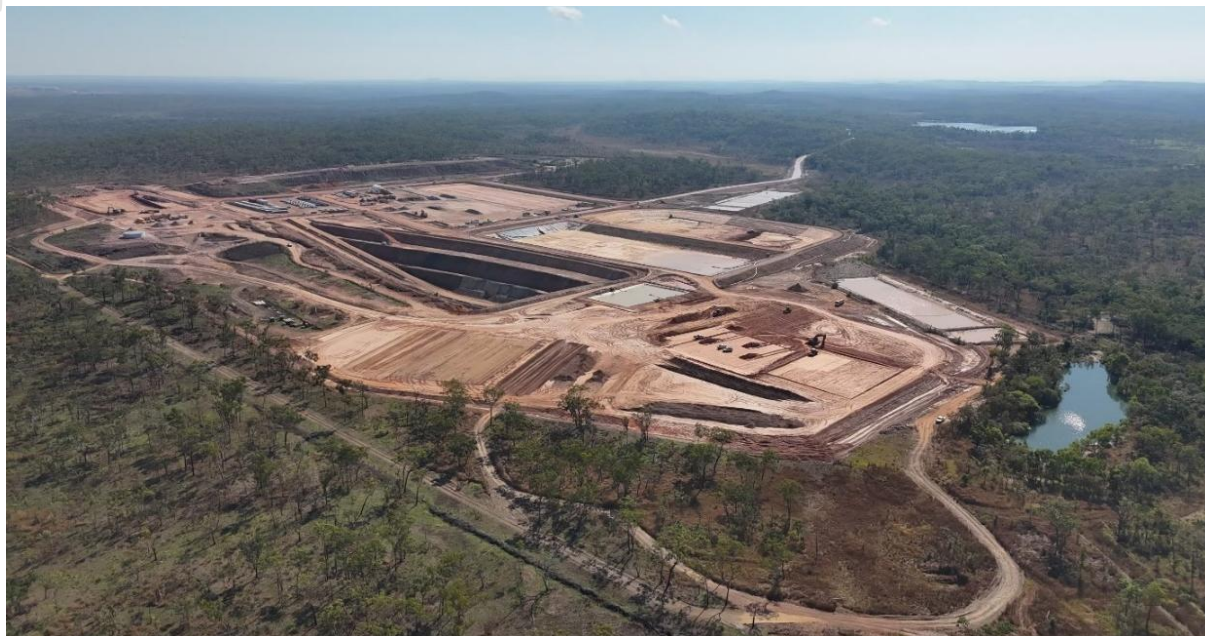
Figure 1: BP33 site overview with preparation of bulk earthworks pads for power station, primary fans and paste plant in foreground
