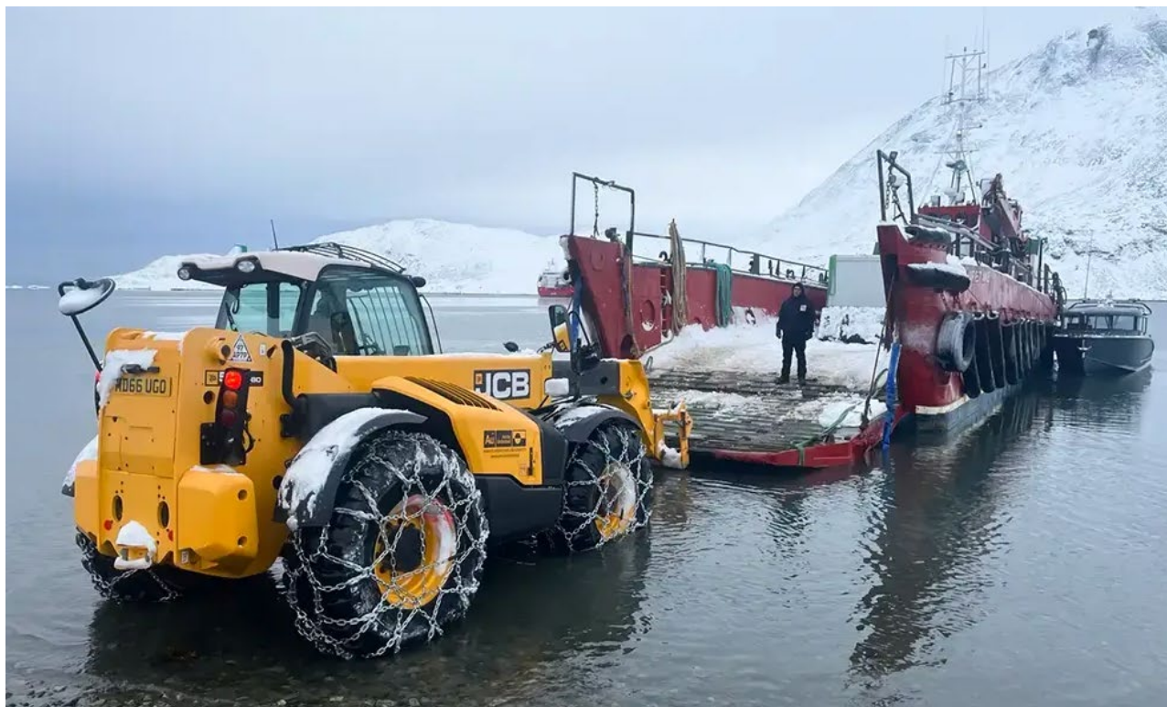
Figure 1. Barge and equipment being mobilised to site.
