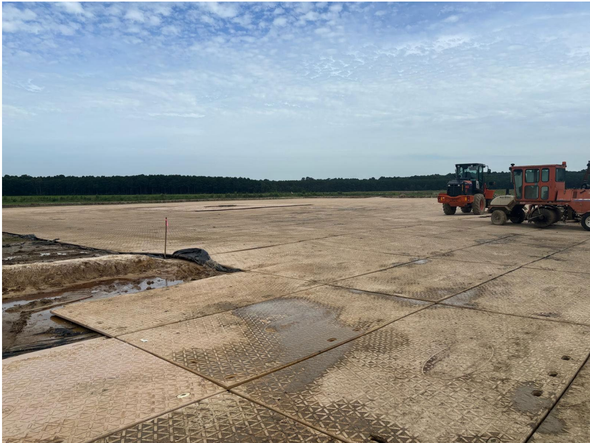
Figure 1: Completed Drill Pad at Zydeco-1 well
