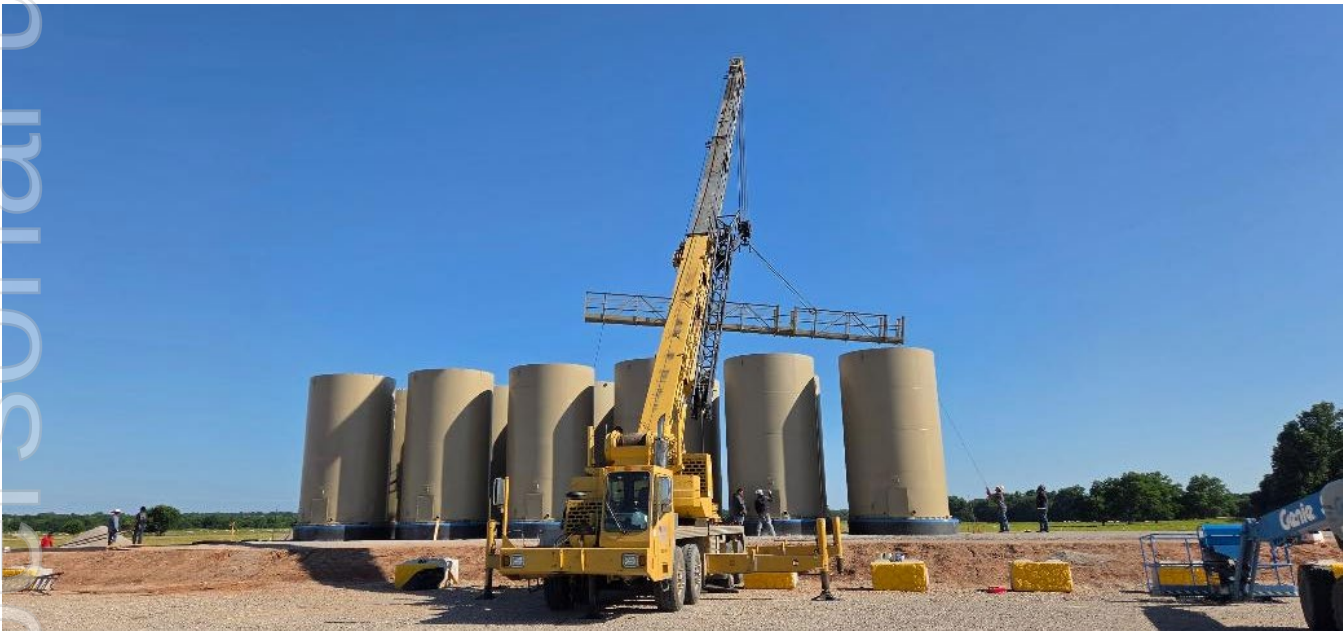
Production facilities under construction at Brookside's Suttles pad in the SWISH AOI, Oklahoma.
