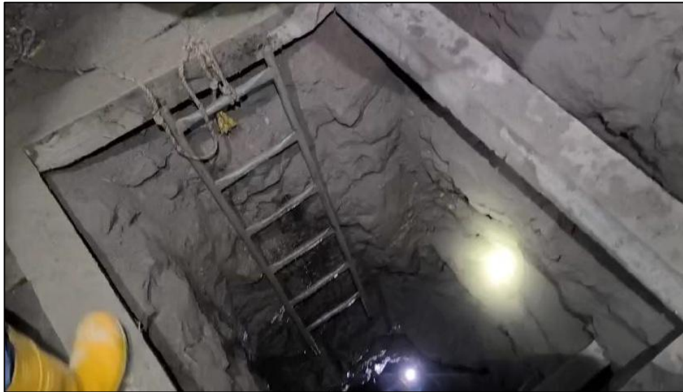
Photo 1: Shaft #2 sinking on Santa Barbara Vein #1.
