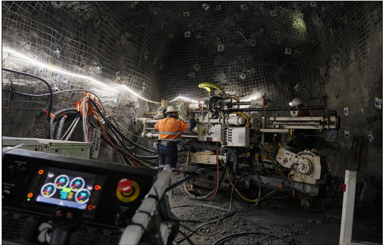
Figure 5: Current underground drilling.
