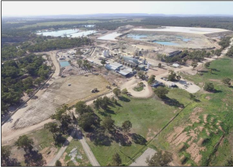
Figure 3: Mineral Hill Processing Plant and overview.
