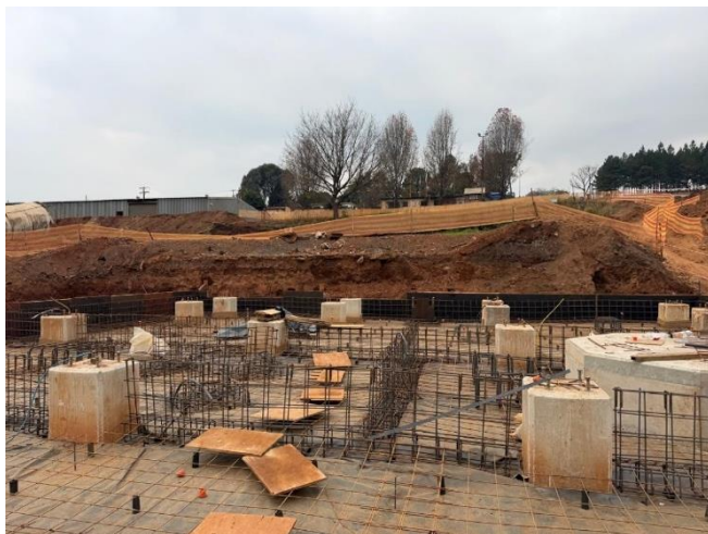
Figure 4: Elution circuit foundations
