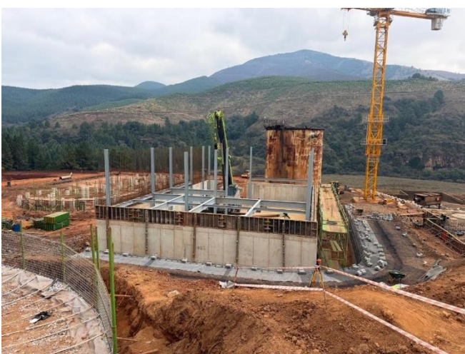
Figure 6: Gold Room construction continues - steel works
