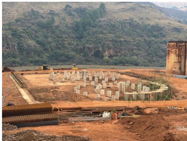
Figure 5: Thickener tank/processing area foundations
