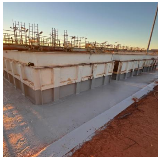
Acid proofing at mixer settlers complete
