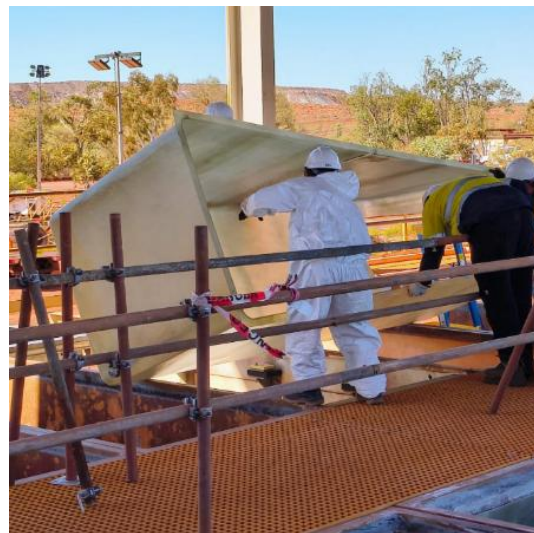
Installing fiberglass inserts for EW cells
