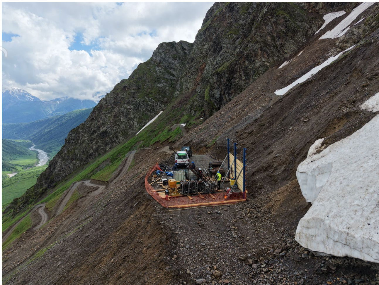
Figure 1 Drill rig on platform at Zopkhito
