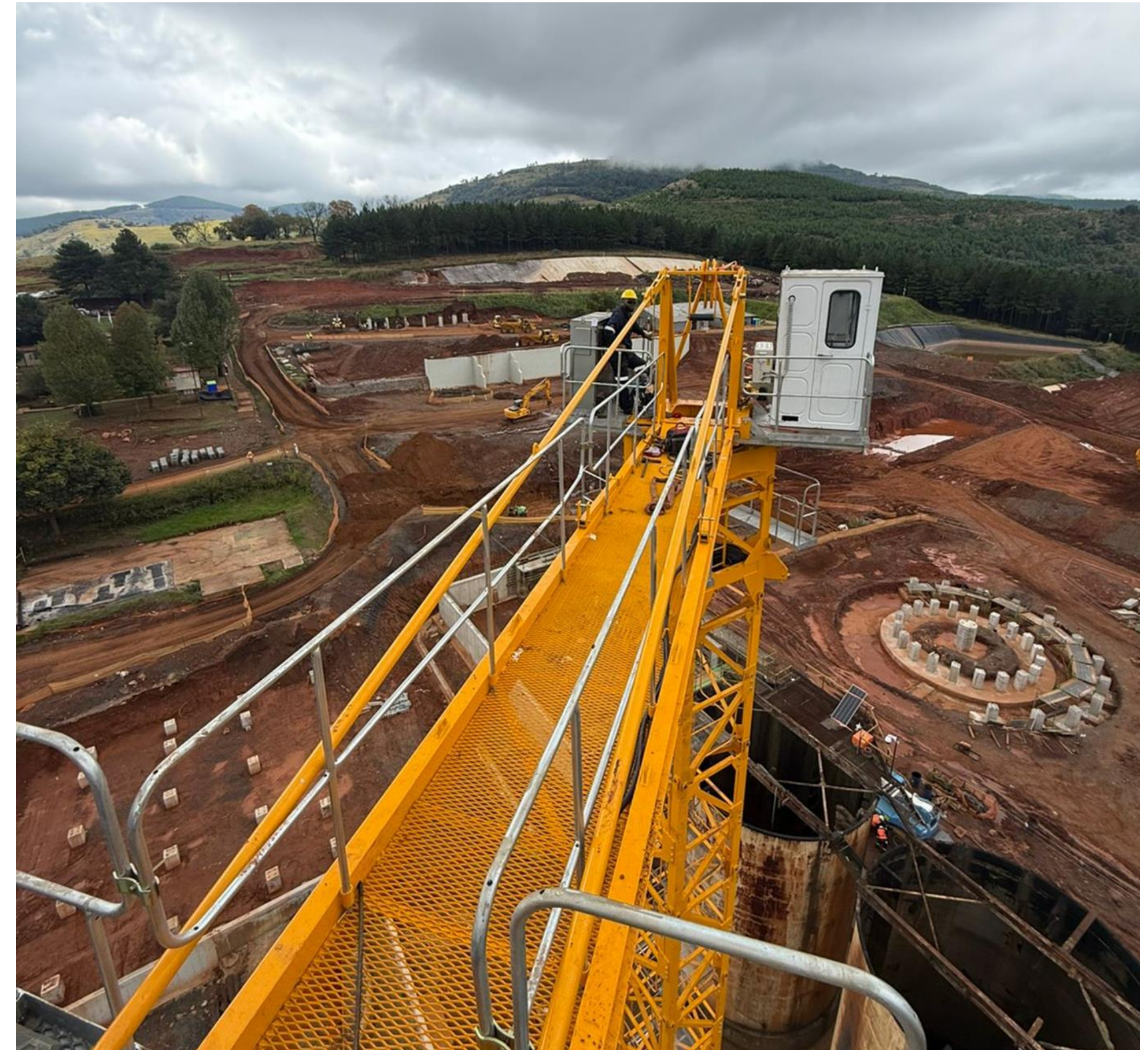
View across TGME Gold Plant site works and construction in progress
