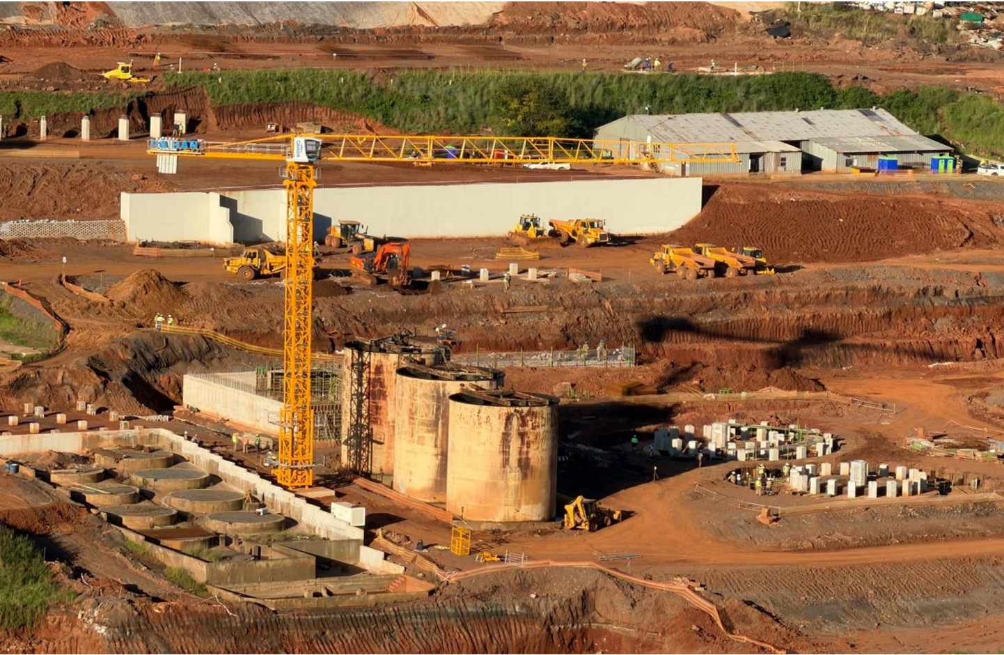
View of TGME construction site looking towards foundation wall for Terrence No.2
