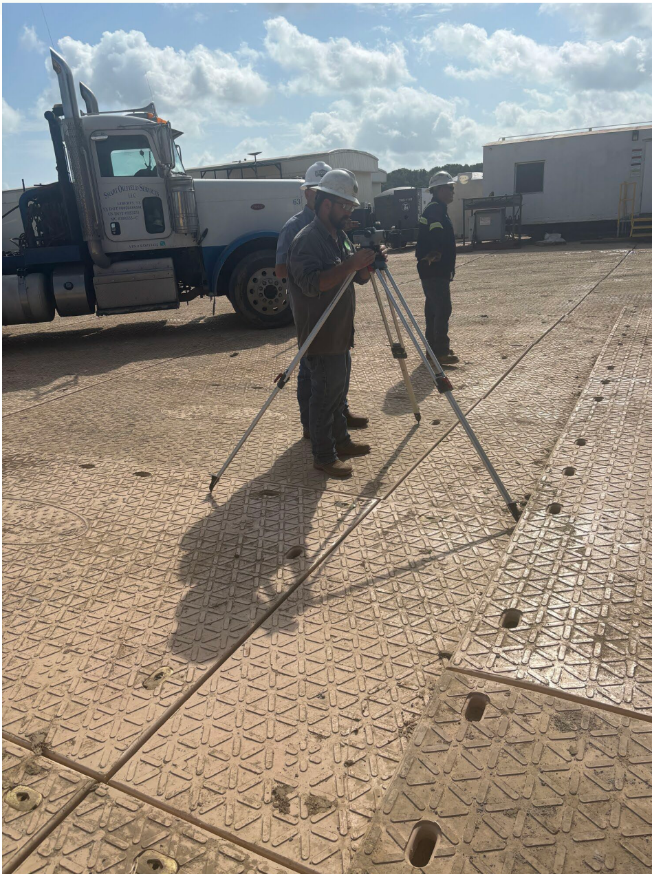
Figure 3: Survey verification of the well centre, conductor location and rig alignment
