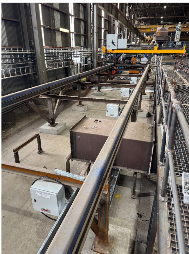
Reduction Furnace local junction boxes & main panel installation progress
