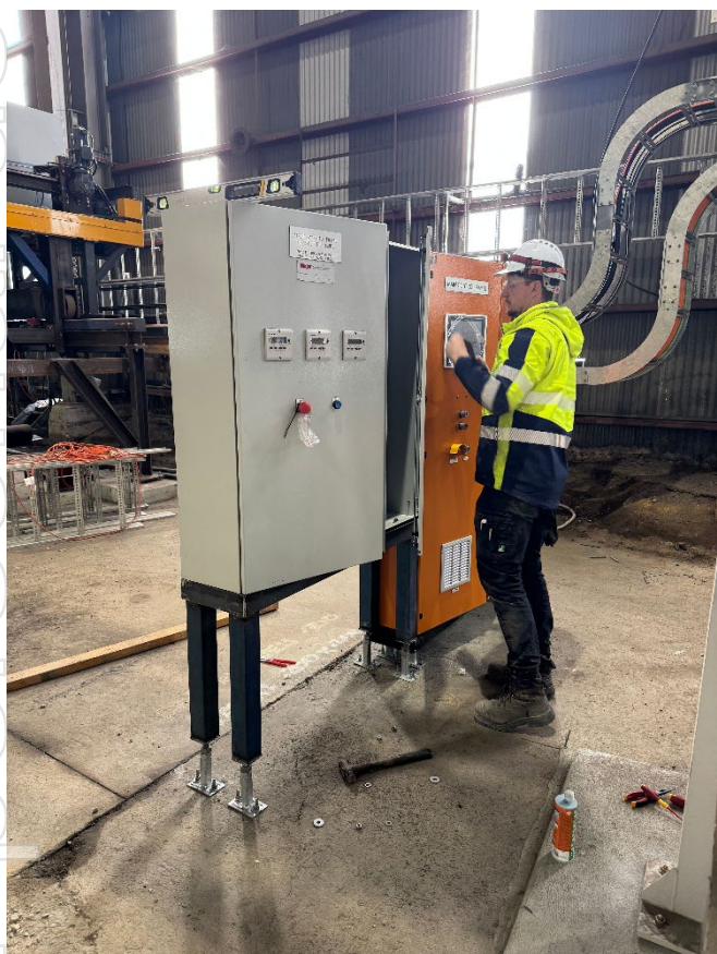
Reduction Furnace local junction boxes & main panel installation progress
