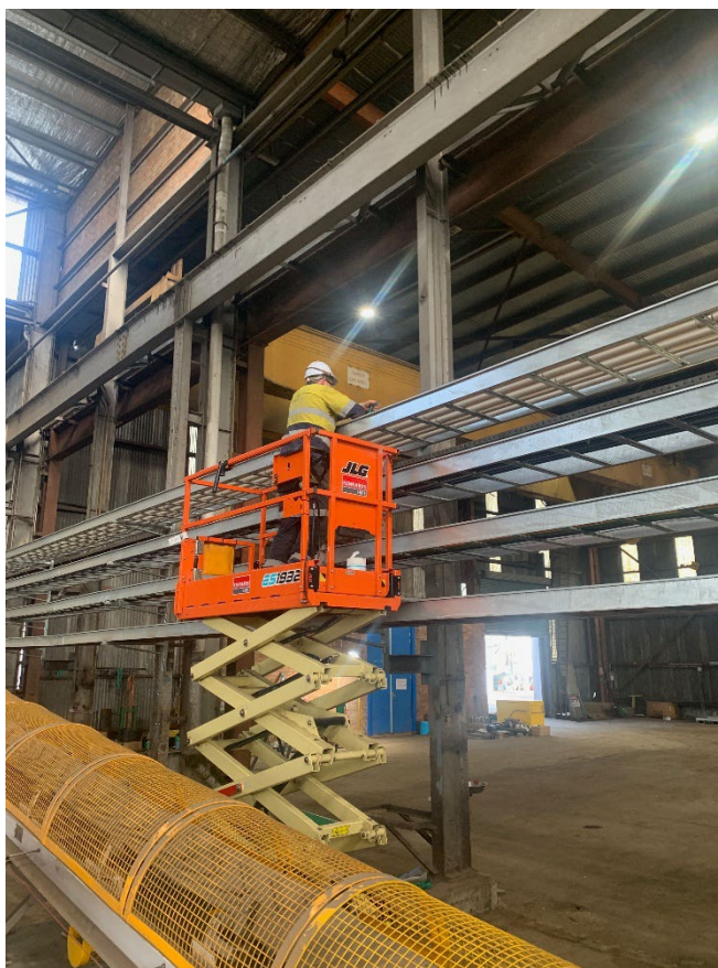
Exhaust stack support fabrication and utility piping and argon supply installation progress
