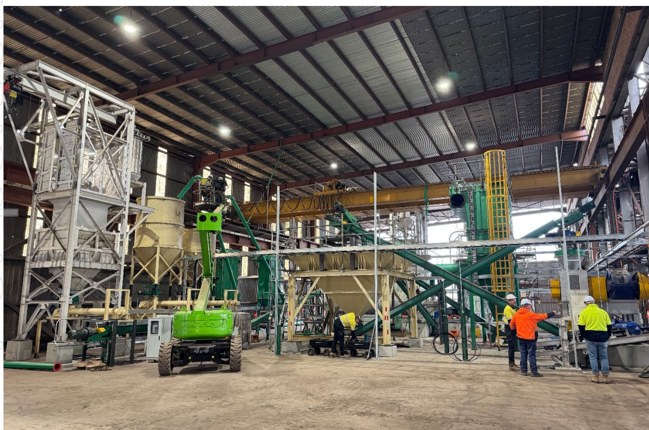
Briquetting area SMP installation progress
