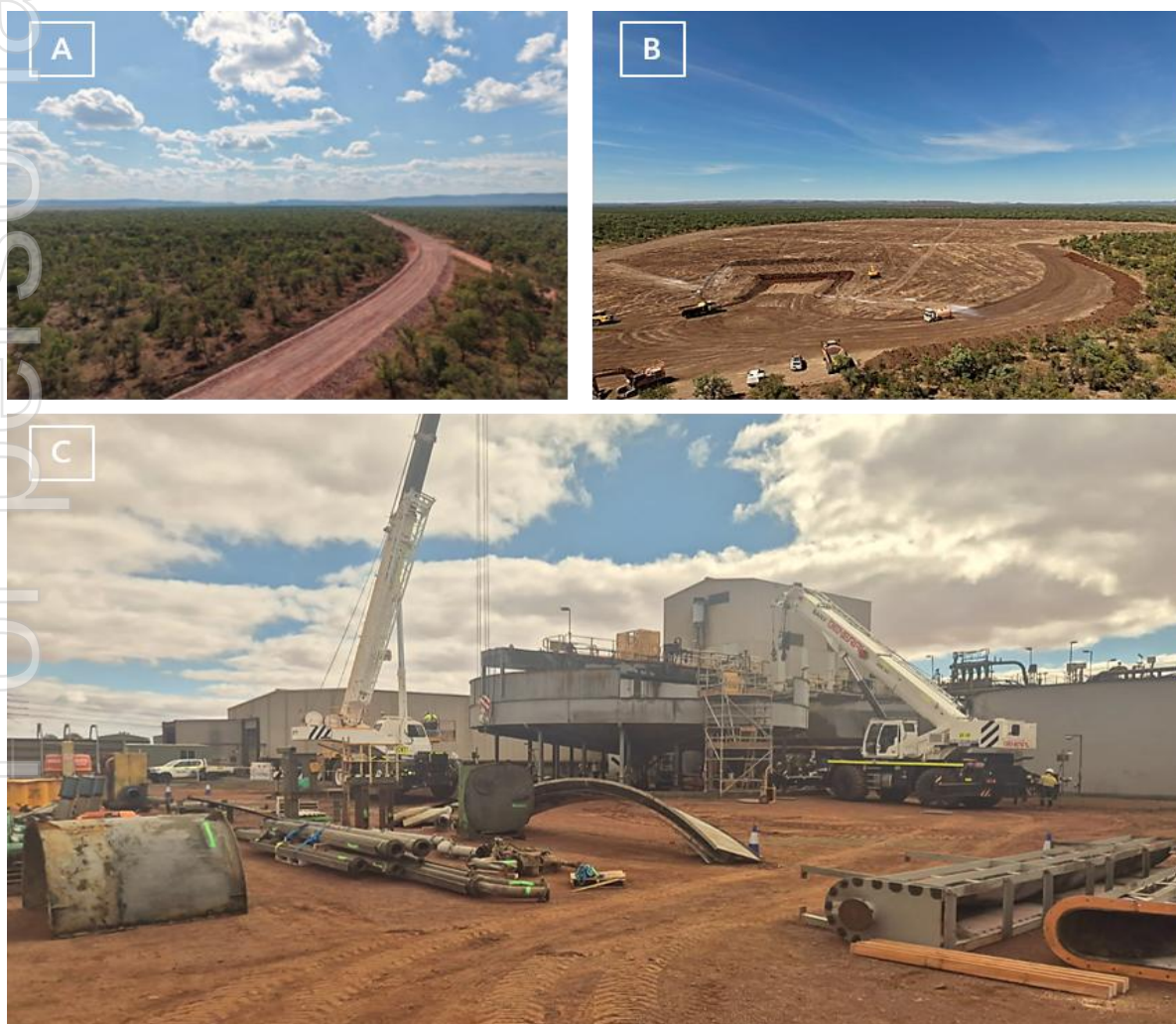
Figure 2: A) All Weather Site Access Road into Sorby Hills. B) Clearing and early mining activities at B-Pit. C) Dismantling activities at DeGrussa.
