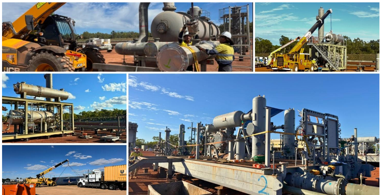
Construction of the Carpentaria Gas Plant
