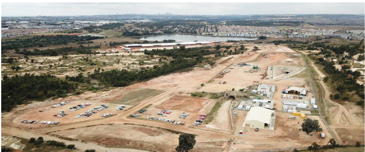
IMAGE 1: AERIAL VIEW OF THE QALA SHALLOWS SURFACE FOOTPRINT AND ONGOING DEVELOPMENT OF SURFACE INFRASTRUCTURE
