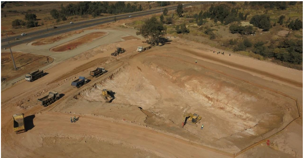
IMAGE 2: TERRACING WORKS ON THE POLLUTION CONTROL DAM
