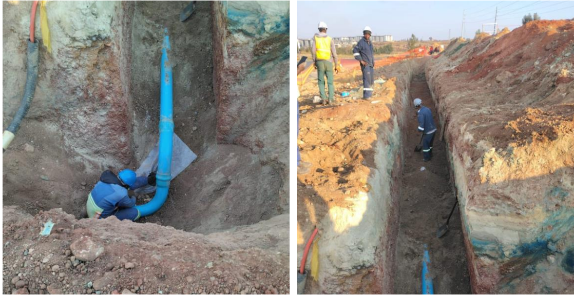
IMAGE 3: INSTALLTION OF POTABLE WATER INFRASTRUCTURE WHICH INCLUDES CONNECTION TO MAINS WATER SUPPLY.
