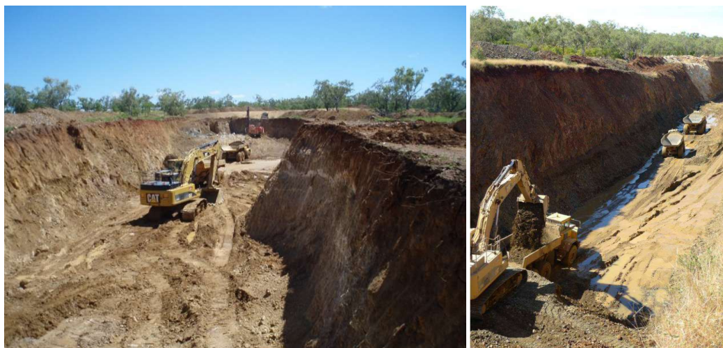
Figure 1: Red Dam pit at end of stage 1 mining in Dec 2010 (left) and Stage 2 mining June 2011 (right)
